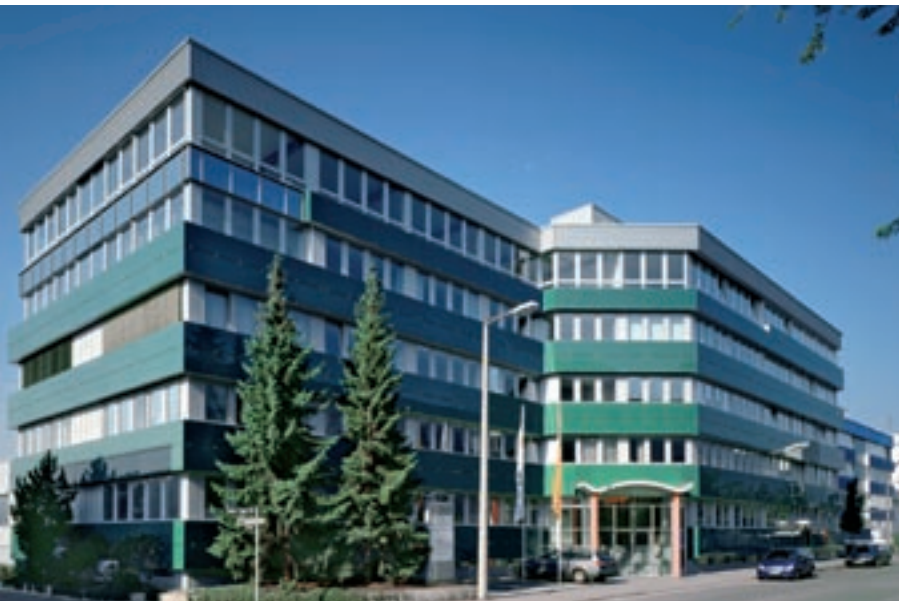
Lapp-Center in Stuttgart
